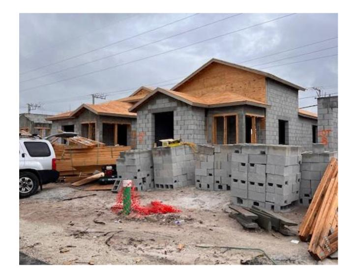
Roof Truss and work and addition of porches
