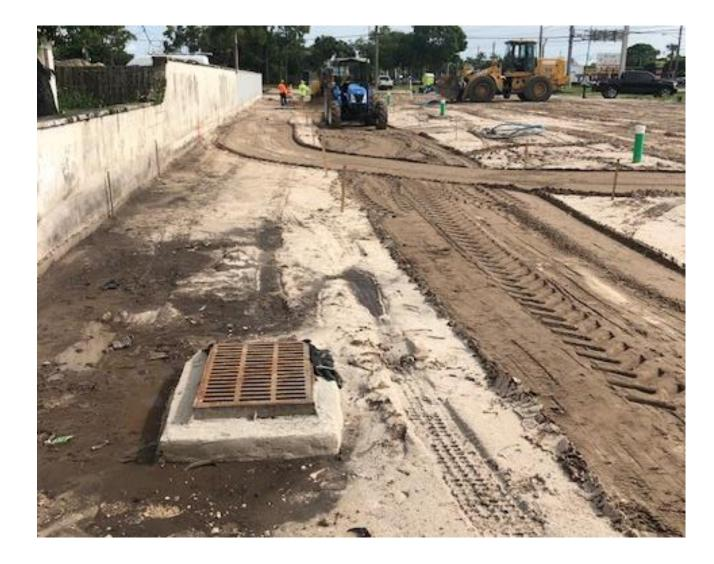
Installation of Road bed and drainage system
