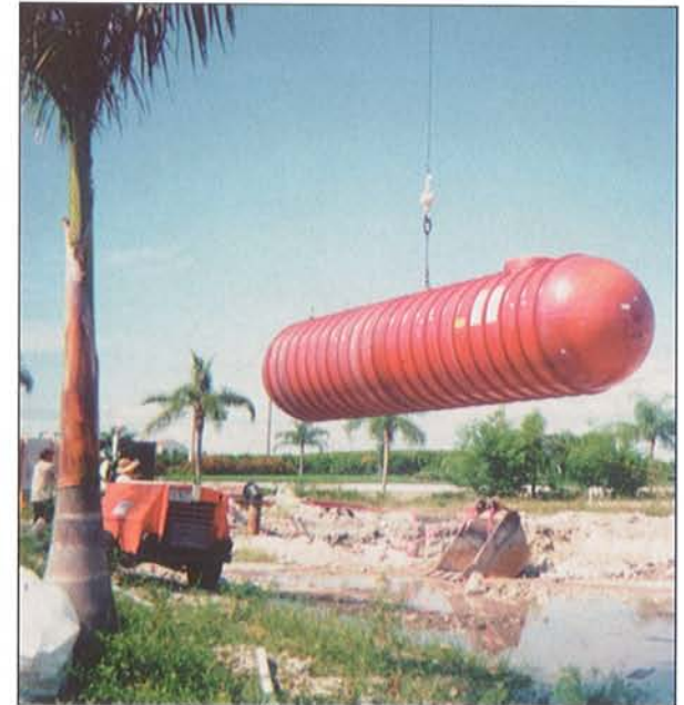
An underground tank is carefully lowered into the excavation.
