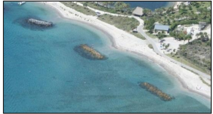
Peanut Island Breakwaters, Palm Beach County, Florida
