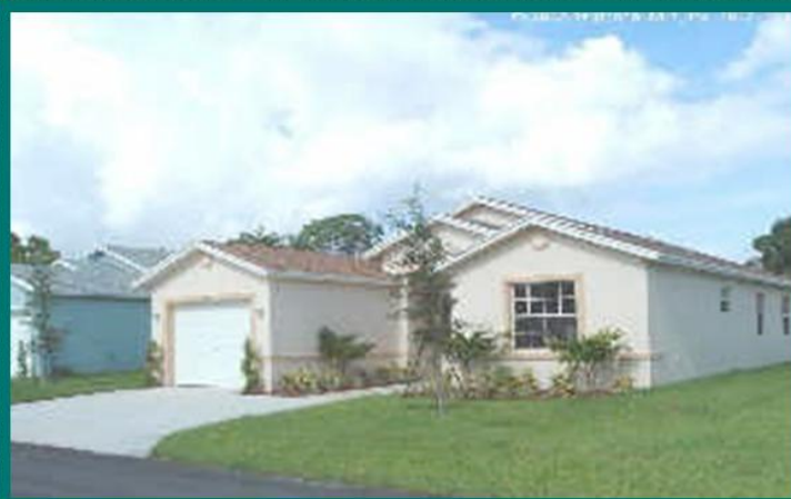
3852 Dale Road & 3864 Dale Road in Palm Springs
