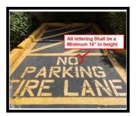
Per the AHJ, any parking space that is required to become a Fire Lane SHALL have diagonal stripes the color of traffic Yellow at a minimum 4" in height, maximum spacing 36", and the words No Parking Fire Lane at a minimum 16" in height located at the front half of the space. The painted lines Shall be Thermoplastic.
