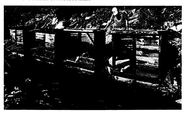
The existing PC 17 culverts have significant holes which allow surface waters from the project area to flow in an unrestricted manner into the western leg of the C-18 Canal. These four culverts will be removed and replaced with two new culverts using NAWCA small grant funding. (Photographer - Harper Carroll, Palm Beach County Department of Environmental Resources Management; no copyright
