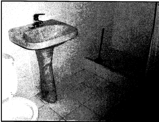
Bathroom In Converted Garage
