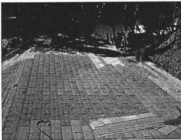
Roof Shingles of different coloring show extent Multiple repairs (NOTE: Newer shingles at top of photo due to tie-in of a building addition not repairs).
