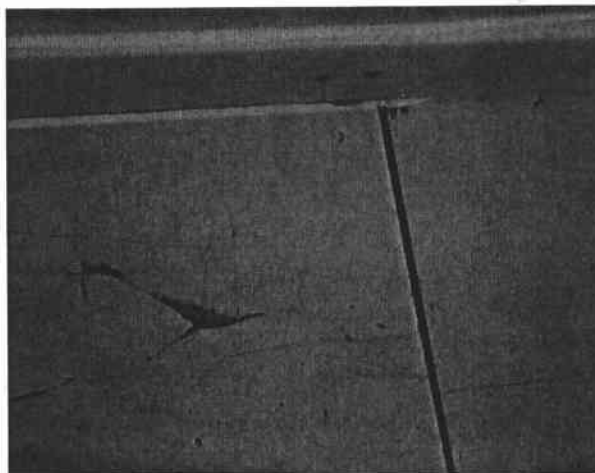
Cracked tiles due to warping floor in the kitchen dishwashing building.
