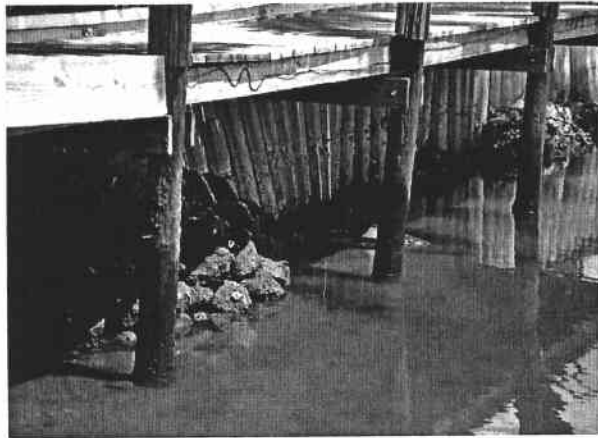
Bowing of The Restaurant site seawall with rocks placed to prevent total failure and washout.
