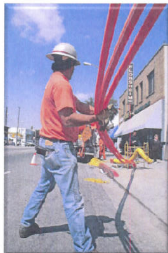
Installing Fiber Optic Cable
