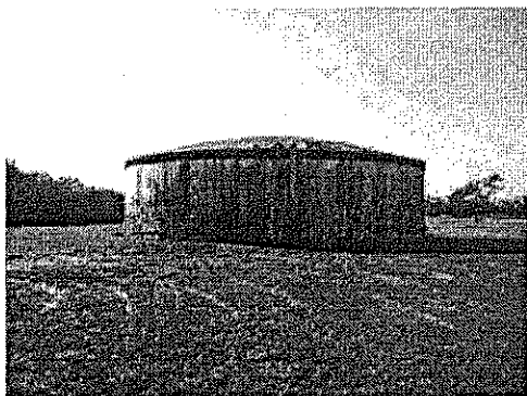
View of the former water holding tank from the north
