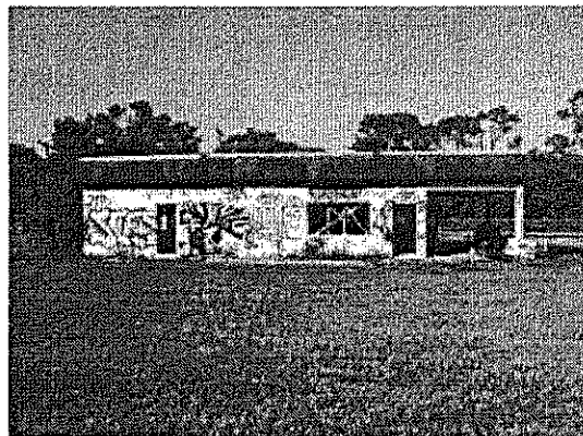
View of the former control building from the east
