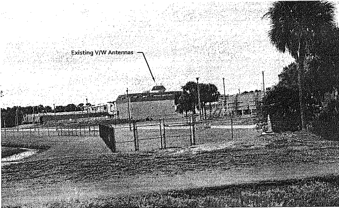
Looking East 1800'± View from Florida's Turnpike taken before installing antenna.
