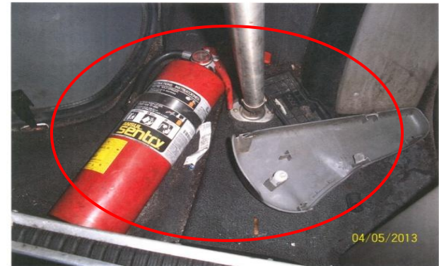
Unsecured extinguisher & electrical covers
