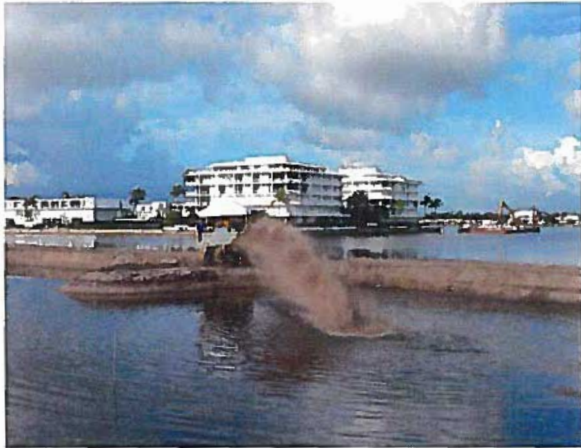
Figure 3. "Sand cannon" in operation for the Ibis Isle Restoration Project (PBCERM)
