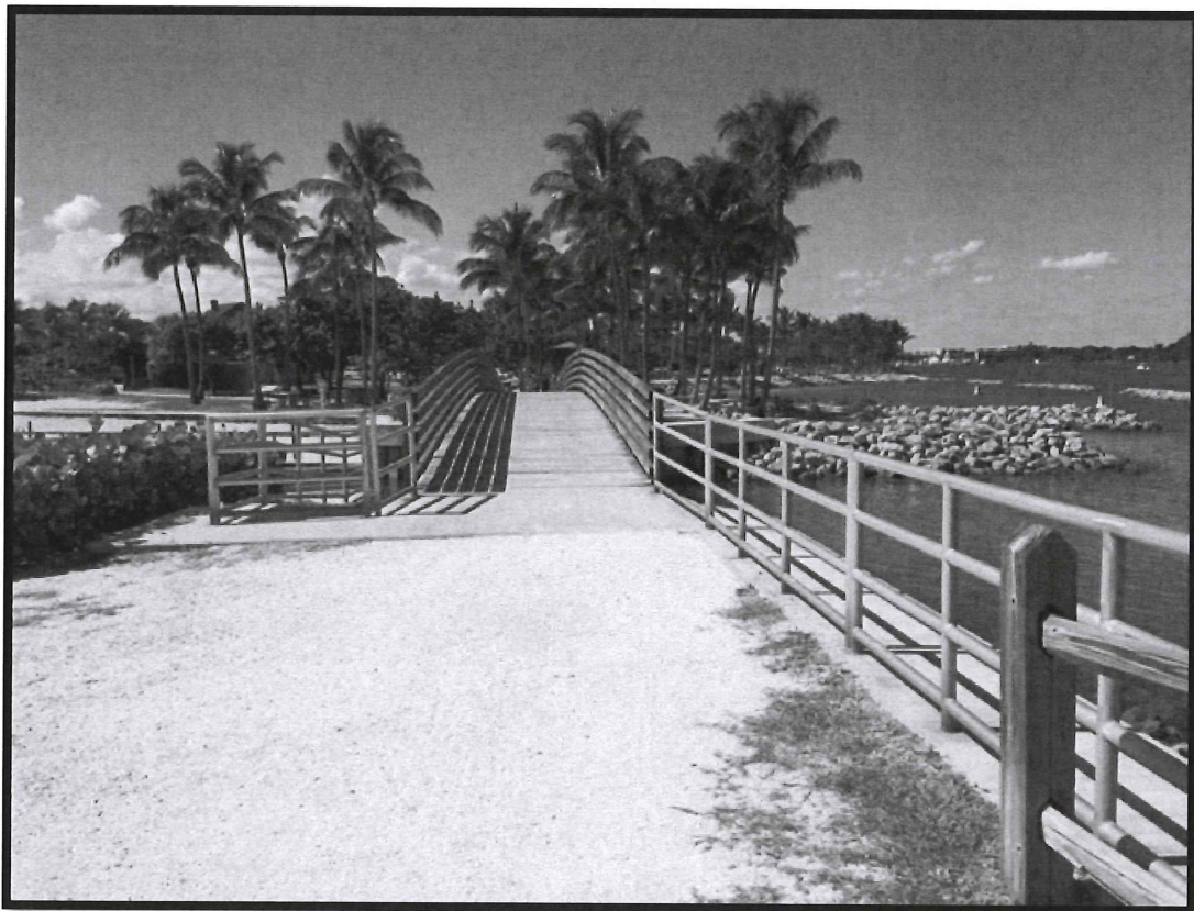
Pedestrian bridge over the tidal creek, renovations include installation of aluminum hand railings, new concrete aprons on approach, modifying bridge slope to adhere to current ADA requirements and replacement of wood decking.
