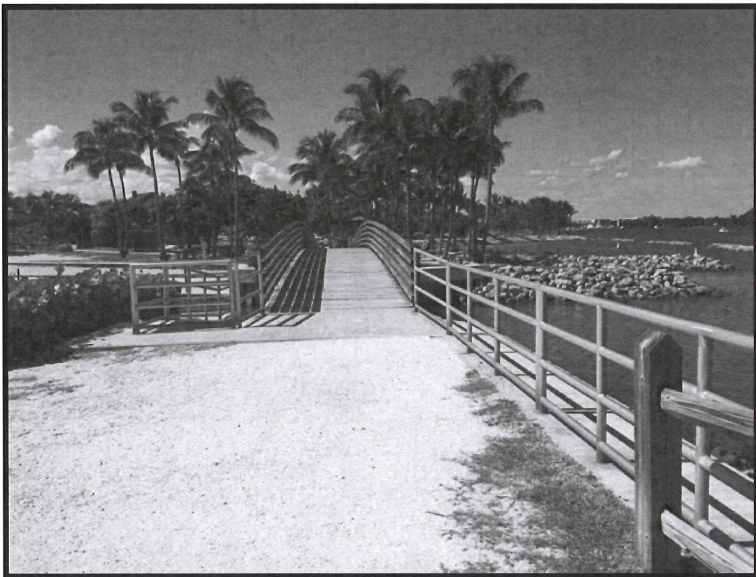
Pedestrian bridge over the tidal creek, renovations include new aluminum hand railings, new concrete aprons on approach, modifying bridge slope to adhere to current ADA standards & replacement of decking.
