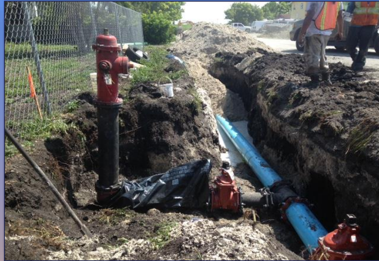
Water Distribution: WM Installation
