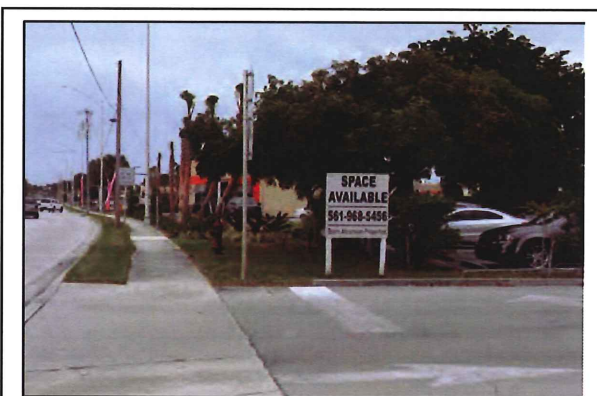
Typical outdated strip commercial along Forest Hill Boulevard in the proposed CRA. Many commercial sites have vacancies and are seeking tenants.
