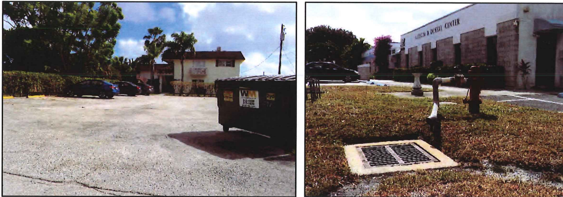
Poor property maintenance and deficient property conditions are a reflection of the declining assessed values in the CRA.
