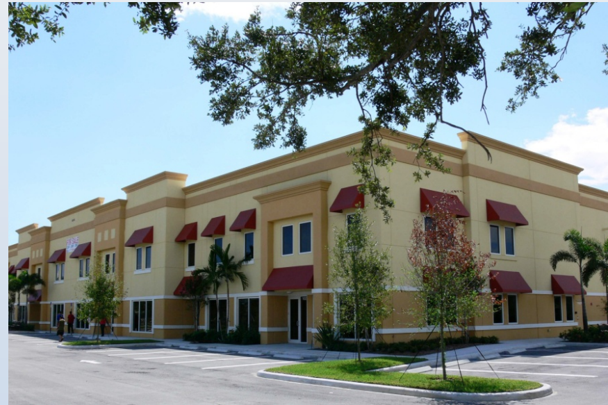
Midpoint Office Warehouse
