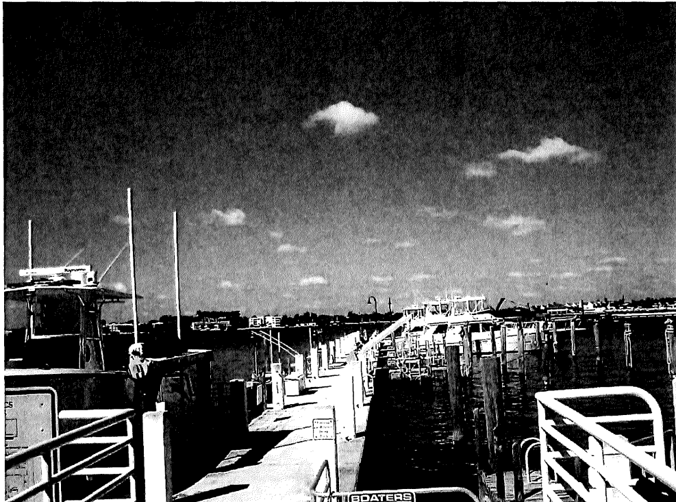
View of marina from bulkhead
