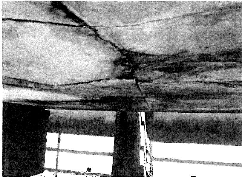
Spalling along the pier
