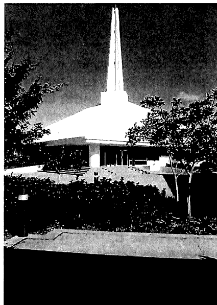
FIRST BAPTIST CHURCH – BOCA RATON FLORIDA.
