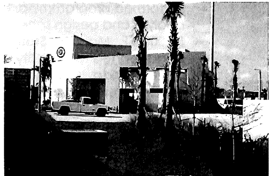
FIRE STATION #31 LAKE WORTH,
