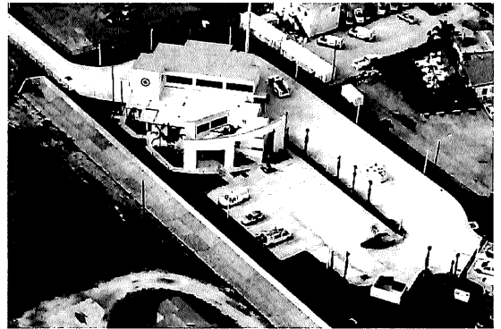
FIRE STATION #31 LAKE WORTH,
