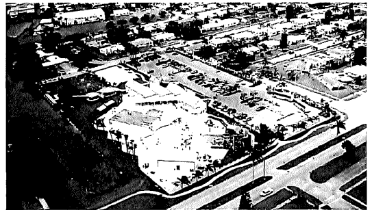
CALYPSO COVE AQUATICS FACILITY
