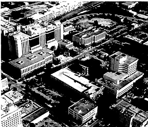
PALM BEACH COUNTY JUDICIAL CENTER COURTHOUSE / STATE ATTORNEY, PUBLIC DEFENDER OFFICE BUILDING RE-GLAZING.
