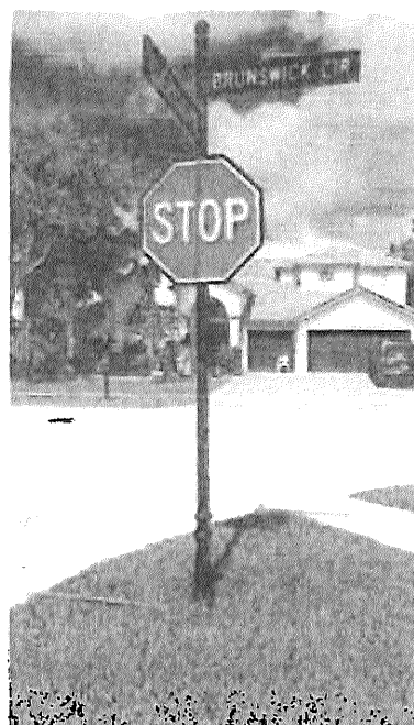
REGULATORY "R1-1:" Sign #14 NOT in compliance with MUTCD
