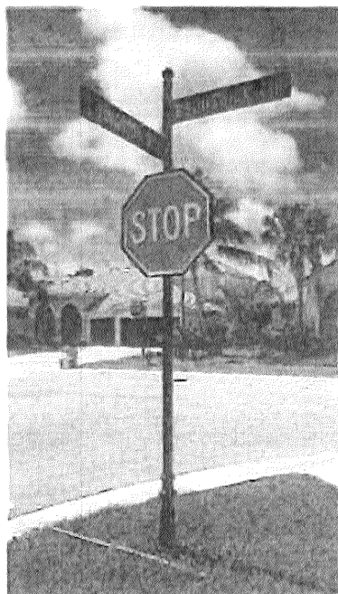
REGULATORY "R1-1:" Sign #16 NOT in compliance with MUTCD
