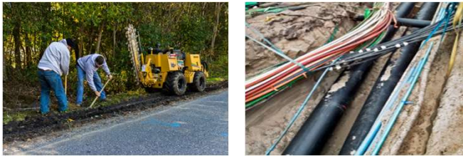
Lay Fiber Optic Cable
