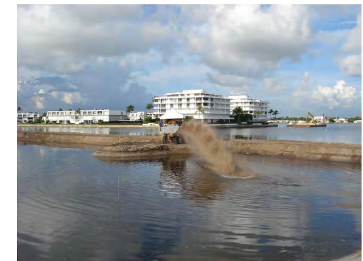
Sand shooter in use at Ibis Isle restoration (Photo credit: PBC-ERM)
