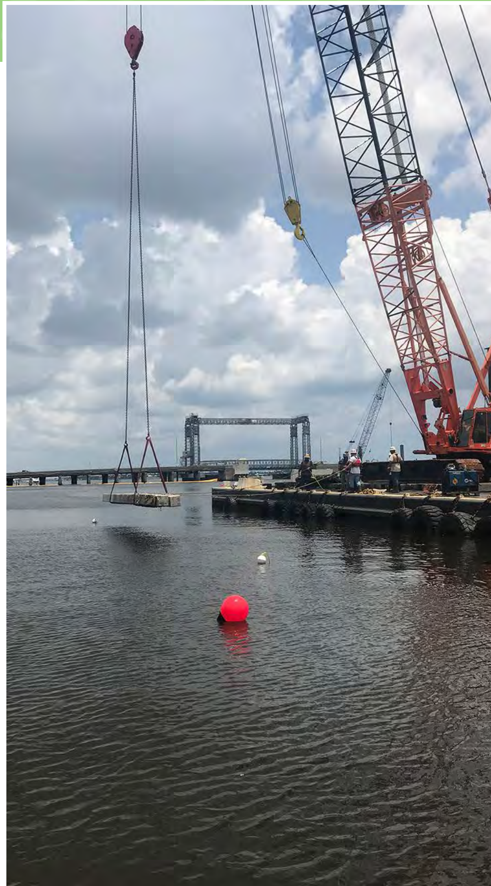
Lowering concrete reef components at Southern Boulevard (Photo credit: PBC-ERM)
