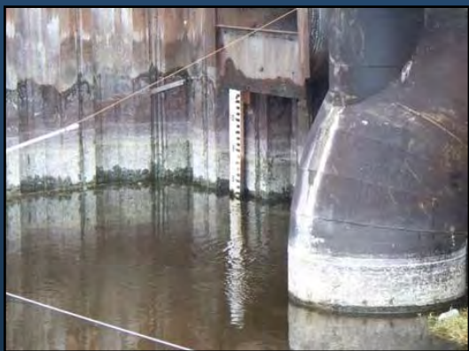
Staff gauge, sets pumping limits
