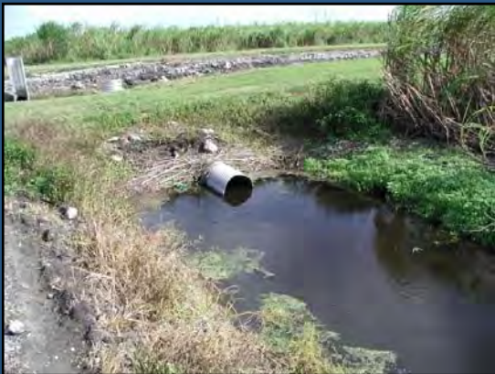
Raised culverts for slower drainage
