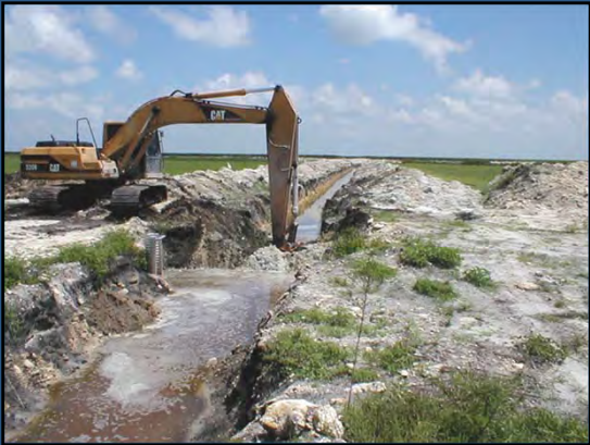
Canal cleaning and capacity improvements
