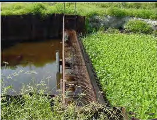
Aquatic weed racks to capture particulates
