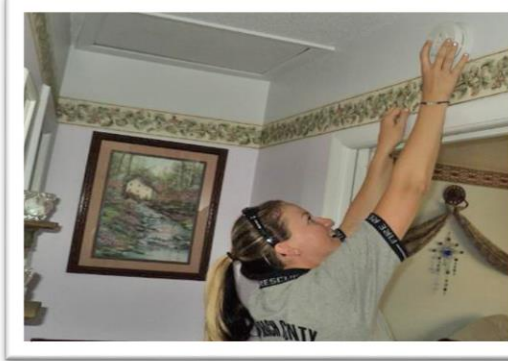
Smoke Detector Installations
