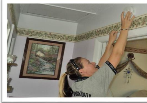
Smoke Detector Installations
