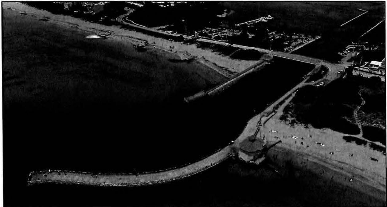
Figure 2. 2016 aerial photograph of South Lake Worth Inlet, facing southwest. Notable features include the north jetty and sand transfer plant, south jetty, T-head groin field, and A1A bridge. Photo courtesy of Palm Beach County.
