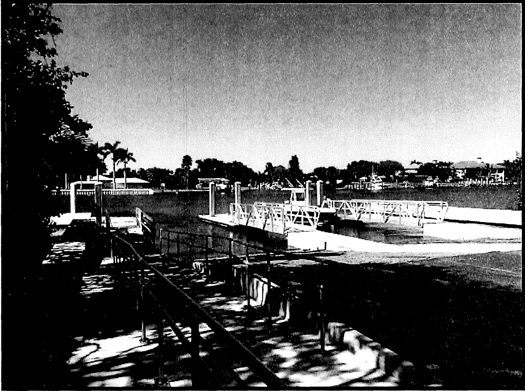
Phase One included three new boat ramps with floating staging docks
