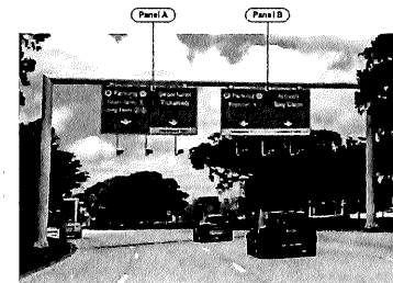
SIGN STRUCTURE RD-08 PANEL A: COVER PORTION OF EXISTING PANEL WITH NEW SIGN PANEL. PANEL B: NO WORK REQUIRED
