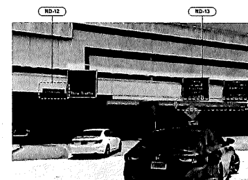
SIGN RD-12 & RD-13 (DEPARTURES LEVEL) RD-12 REMOVE EXISTING SIGN PANEL AND REPLACE WITH NEW SIGN PANEL. RD-13 ADD NEW SIGN PANEL BELOW EXISTING PANELS.
