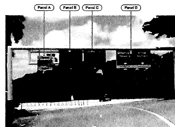
SIGN STRUCTURE RD-10 PANEL A: REMOVE EXISTING SIGN PANEL AND REPLACE WITH NEW SIGN PANEL. EXISTING ADVANCE WARNING SYSTEM ASSOCIATED WITH PANEL A TO BE REMOVED. DEVOUGH EXISTING WIRELESS RECEIVER, ANTENNA AND REMOVE CONDUCTORS ACCORDINGLY. EXISTING SIGN LIGHTING SYSTEM SHALL REMAIN. PANEL B: NO WORK REQUIRED. PANEL C: NO WORK REQUIRED. PANEL D: NO WORK REQUIRED.
