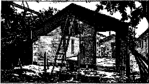
Project in progress at 127 South F Street
