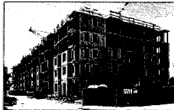
Progress of The Bohemian – South East Coast Street at Lake Avenue
