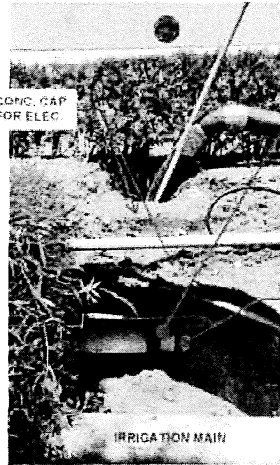
SUSPECTED 6" CHWS, UNDER CONC. CAP
