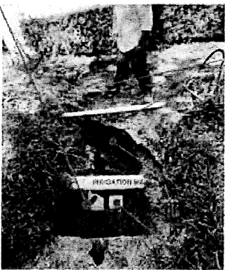
SUSPECTED 6" CHWS, UNDER CONC. CAP
