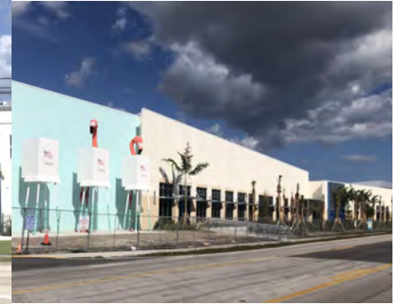
Palm Beach County Supervisor of Elections Facility (Cherry Road)
