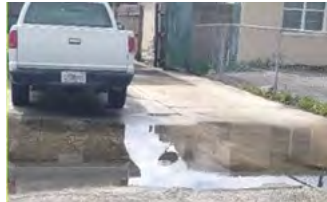
Existing conditions - no sidewalks, no street lighting (above) & (right) flooding in swales due to poor drainage
