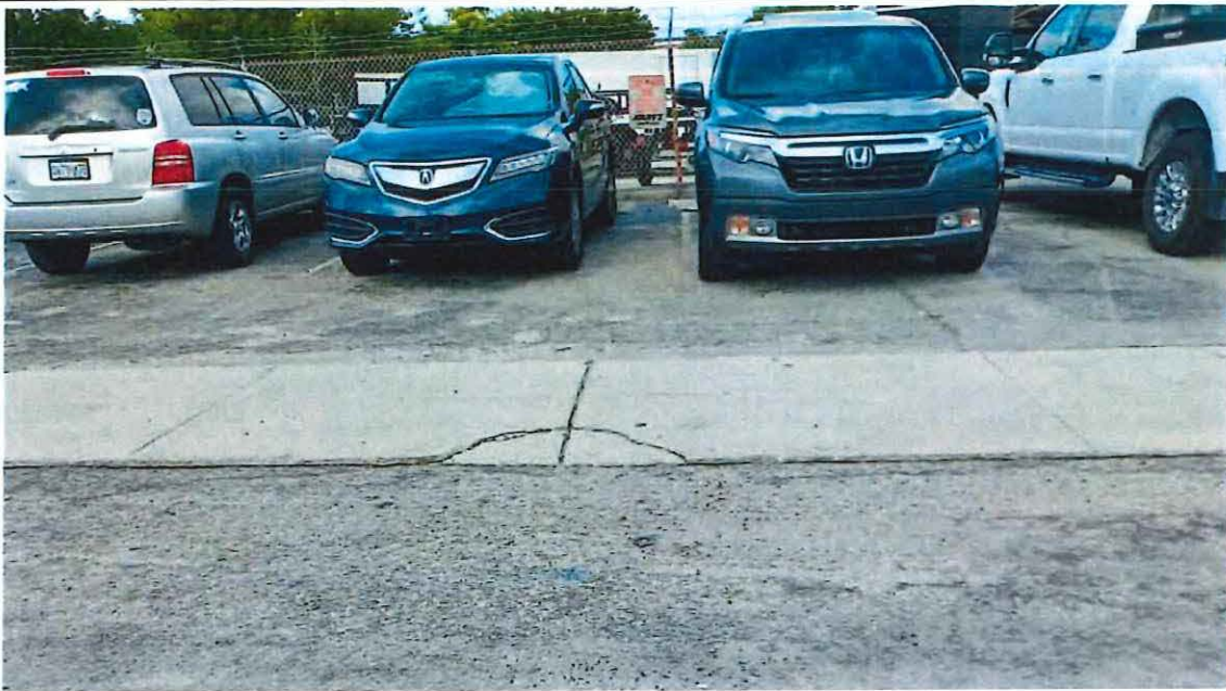
Photo: 10th Court cracked sidewalk showed unsafe conditions
