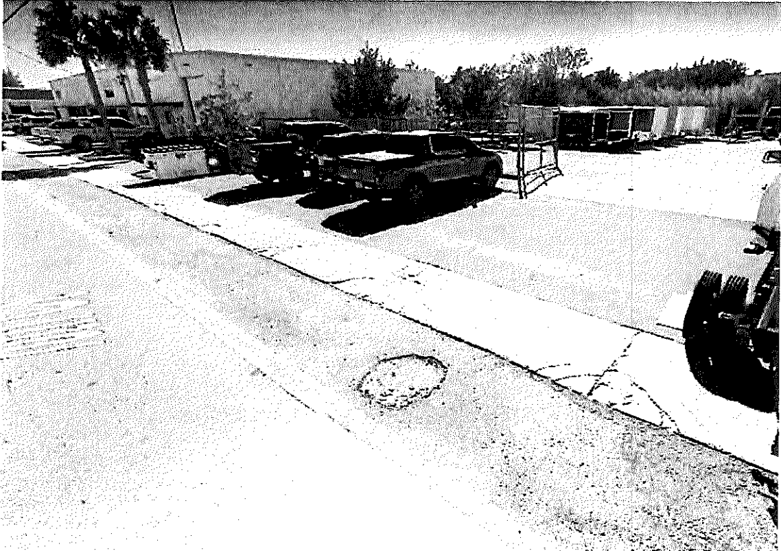
Photo: 10th Court holes in asphalt and cracked sidewalk showed unsafe conditions
