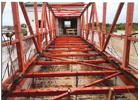
Pedestrian Bridge Rehabilitation
