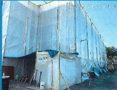
From left: Historic Roosevelt Full Service Adult Education Center gymnasium building before lead paint abatement; preparation of lead paint abatement; abatement process completed
