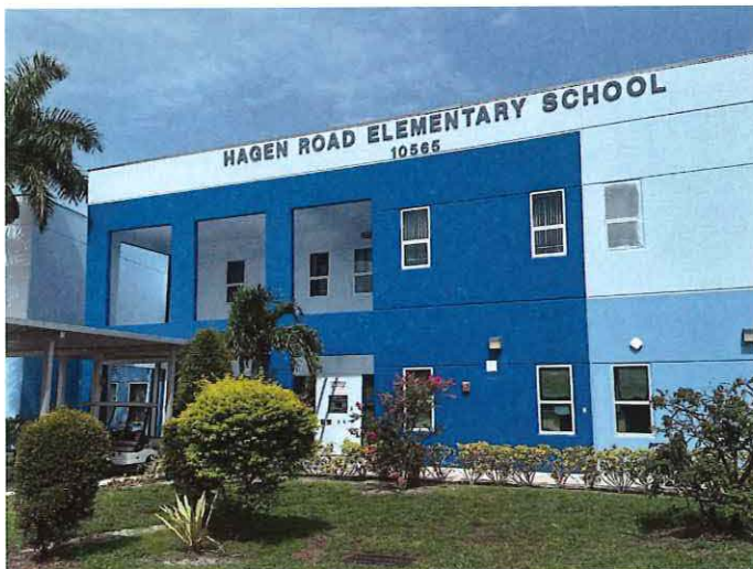
Fresh exterior paint at Hagen Road ES
