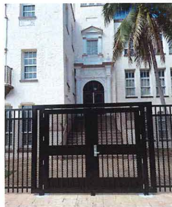
Internal security gate that leads to the single point of entry at Alexander W. Dreyfoos SOA
