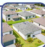
Carver Square Workforce Housing Construction 2023
