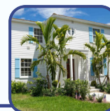
Renovation of Historic Home (Wellbrock House) as CRA Offices 2022
