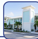
98 NW 5th Avenue Renovation 2023
