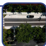
NE 3rd Street/NE 3rd Avenue Alley Improvements 2022
