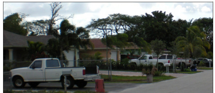
Intact and healthy single family residential neighborhood along Lake Worth Road. These are the neighborhoods the PRAs are to serve.
