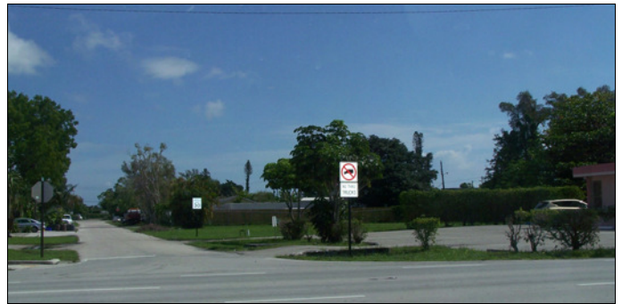
Typical secondary street servicing single family residential homes from Lake Worth Road.
