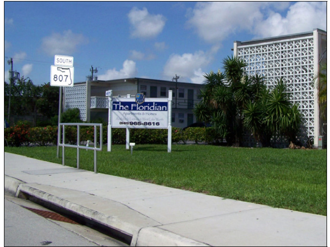
An existing rental apartment along Congress Ave.
