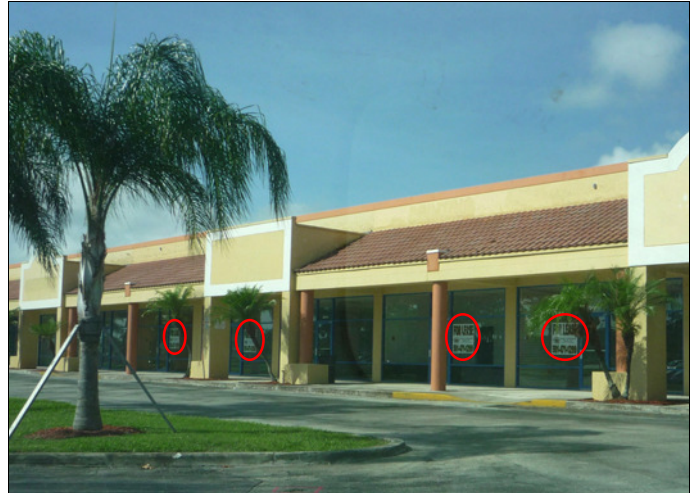
A dated, declining shopping center advertises multiple storefronts available for lease.
