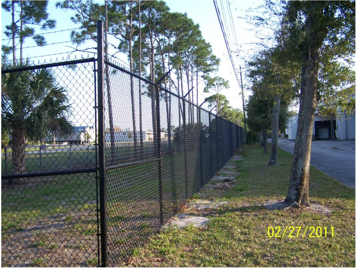
Figure 4 photo of existing landscaping and fence to remain
