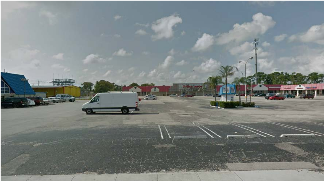
8.c - View from Lake Worth Road into Shopping Center
