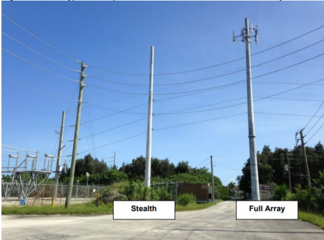
Figure 4.B.9.D – Typical Examples of Electrical Transmission Poles or Utility Structures
